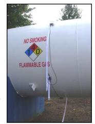
tank. Continue gently pulling the Satellite Box up the tank until the slack is removed from the Satellite Box cable, or until the Satellite box is at the desired location near the top of the tank. **Do not pull hard enough to move the Communication Box and Sensor**. If there is any slack left in the Satellite Box cable, coil the excess cable and secure with a cable tie wrap to remove the slack.
